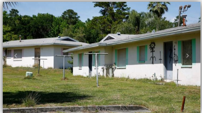
LUIS SANTANA | Times --Buildings that once housed low-income families in Brooksville at Hillside Estates have been abandoned for years. At the urging of the U.S. Department of Housing and Urban Development, the Brooksville Housing Authority recently advertised for proposals to take over the site.
